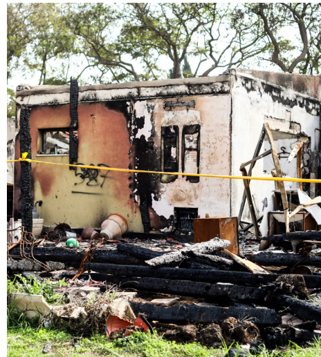
A home destroyed by fire in Kibbutz Kfar Aza.
